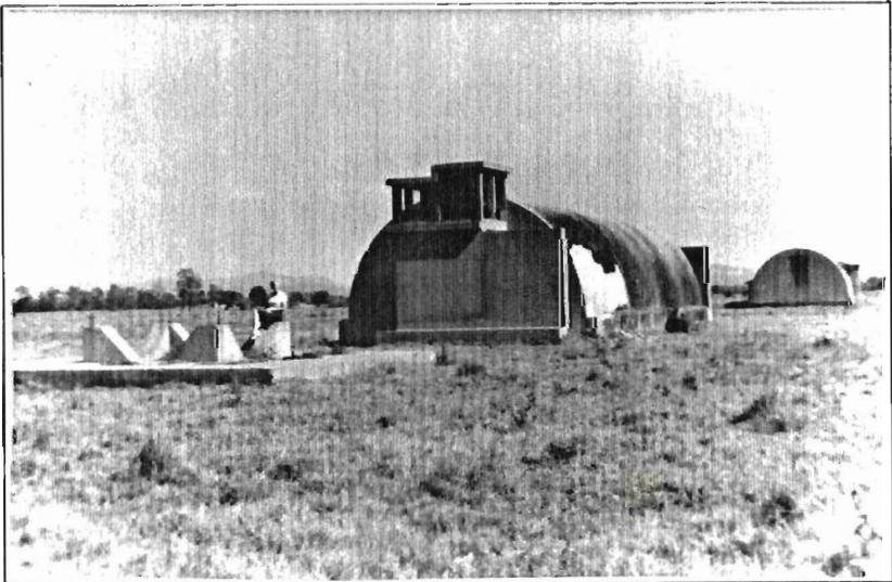
Below : Ash Island 1980. The remains of the concrete igloos, with the base of the RWG aerial in the foreground. These rooms were built in 1943 to an English design for underground operations.
