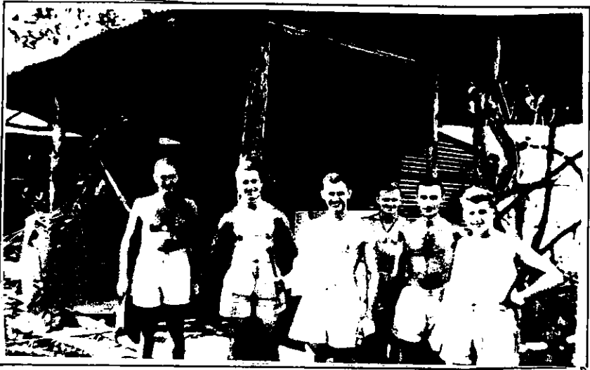
132 RS. Building the new camp at Knuckey's where the Doover was located. Ron Young, Larrie Matters, Harry Samblebe, (Sam), Bill Goodman, Roy Cruickshank, Ron Beestey.
